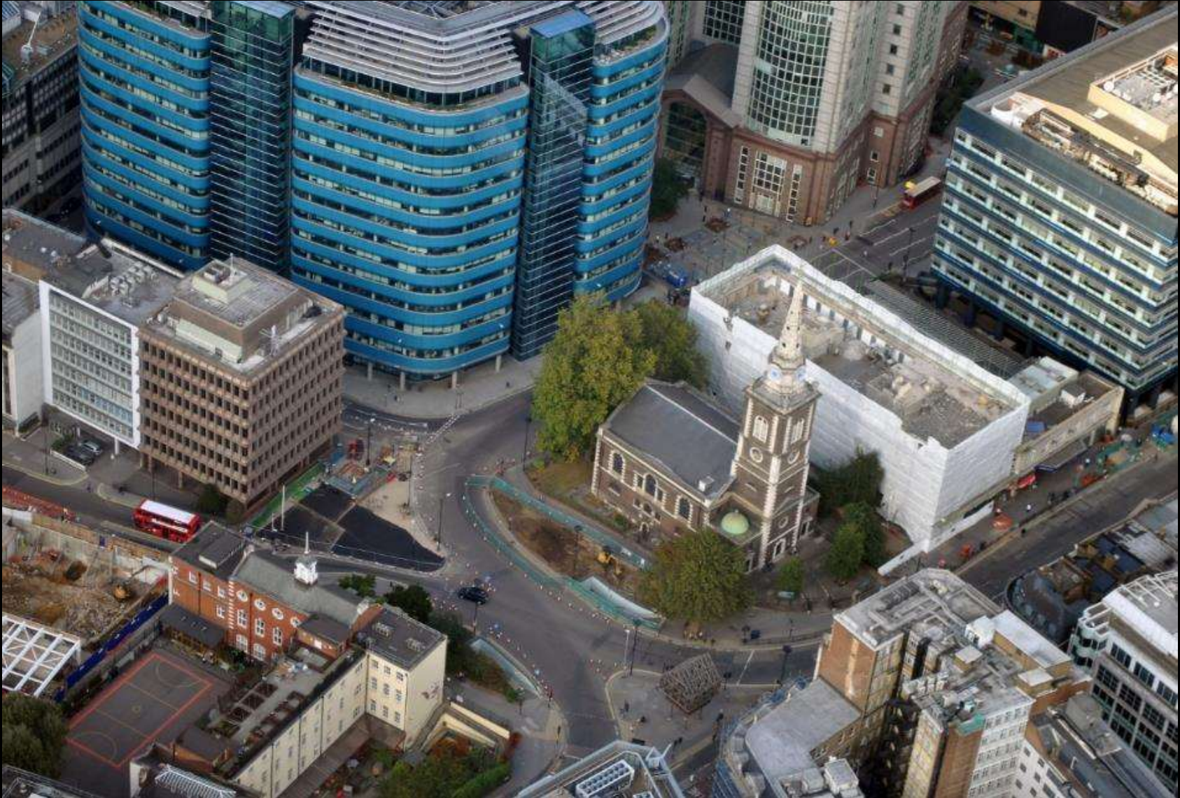
Aerial photograph of Aldgate Gyratory (before)
